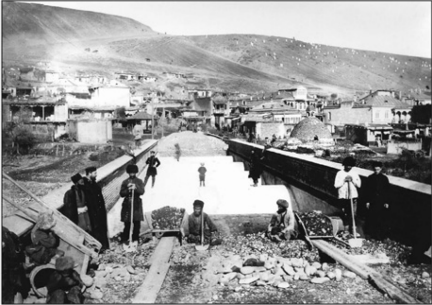
Guba, Construction of a bridge over the Gudiyal-Chay River, 1907
